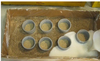
InstaGrout is mixed and poured
