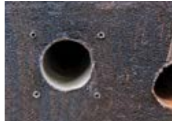
Core drill and pilot holes
