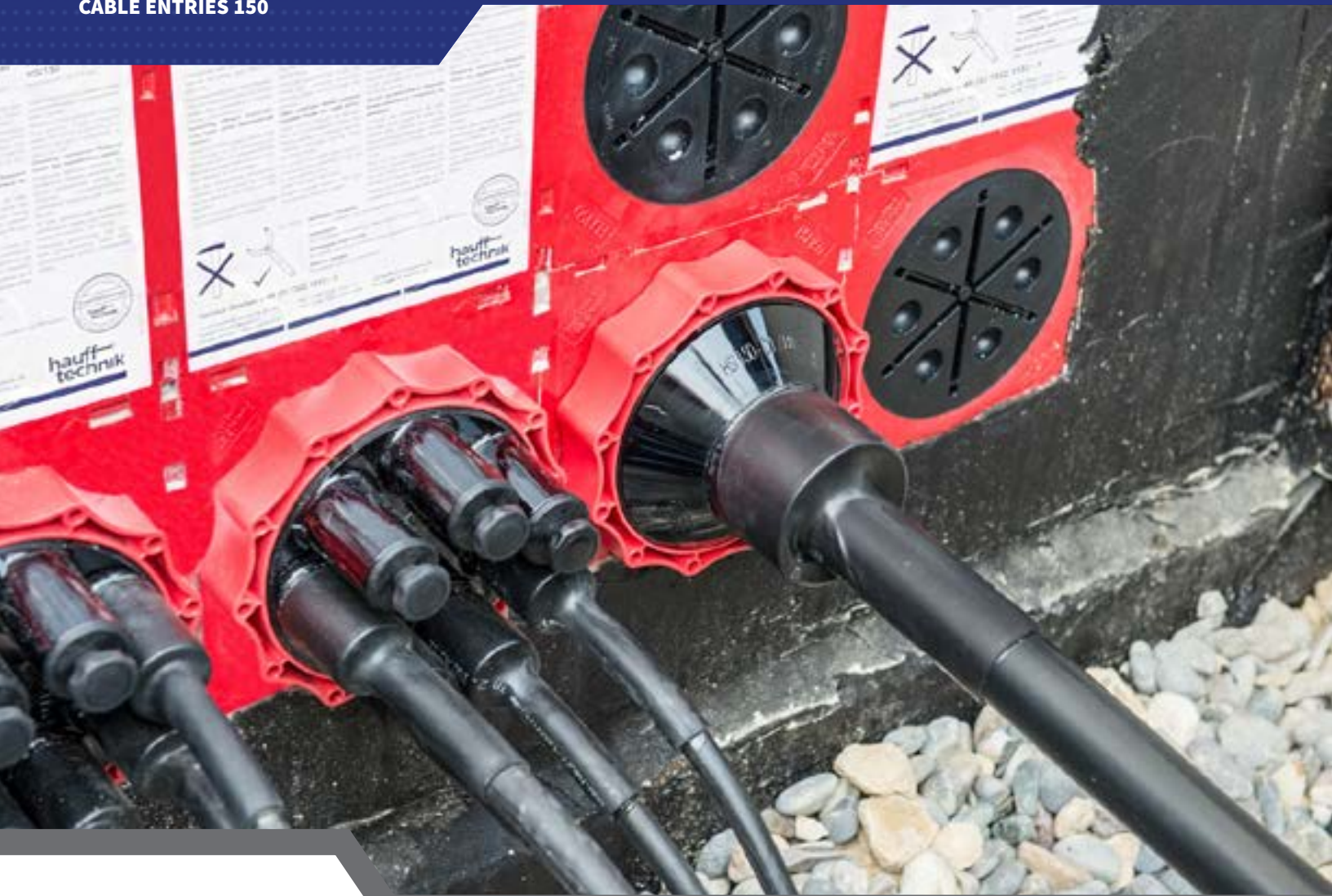
Pictured: Various heat shrink system cover cable seals
