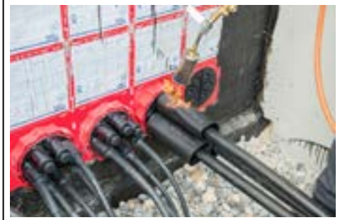
Applying heat to the heat shrink.
