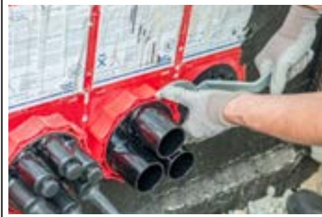
Securing the system cover.
