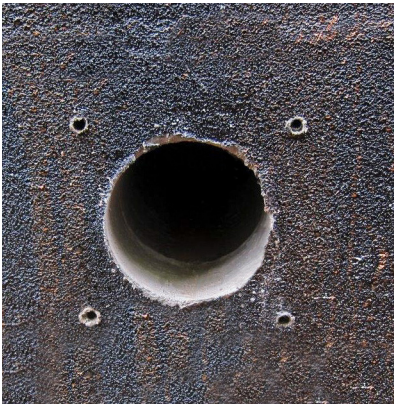
Core drill and pilot holes.
