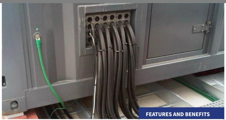
The Optimum Sealing Solution for Multiple Cables Entering Prefabricated Containers or Substation Trenches
