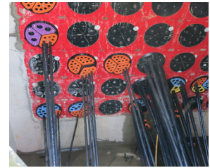
Wall inserts fitted with SEGMENTOS.
