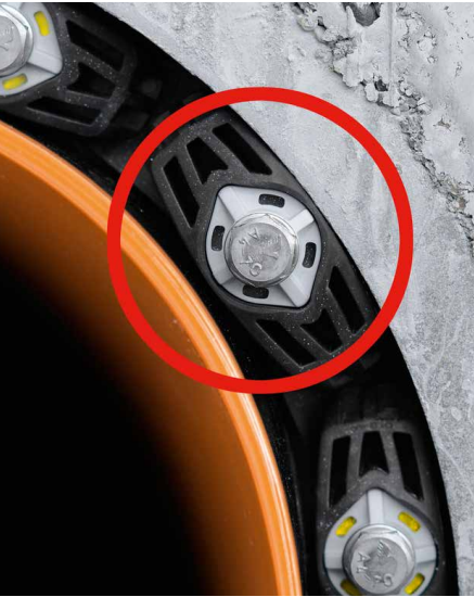
PGKD 400 – tightening of segments
