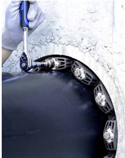
PGKD 400 – tightening of segments
